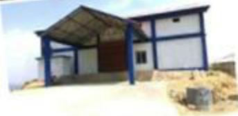
Lungpho Godown Capacity - 352 MT Amount : Rs. 1,25,55,620.00 Under DCSO Kolasib
